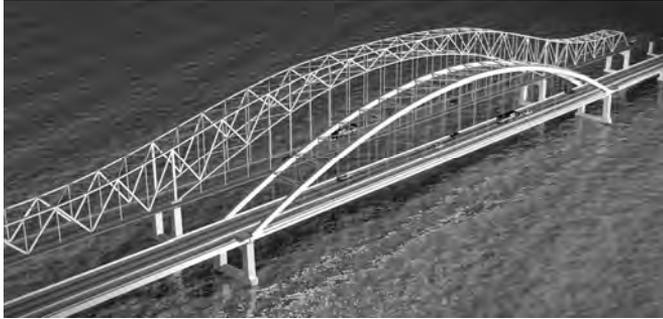
design team and the aesthetic criteria were ranked by the PCC team. The two scores for each alternate were then added together to determine the composite score. The tied arch with lateral x-bracing received the highest composite score and was selected as the final bridge type.
