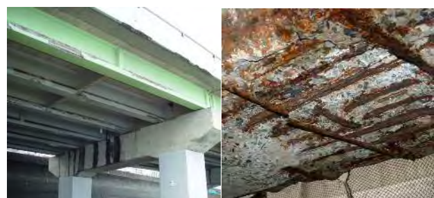
[a] PC I-girder penetrated substantial chloride ion
