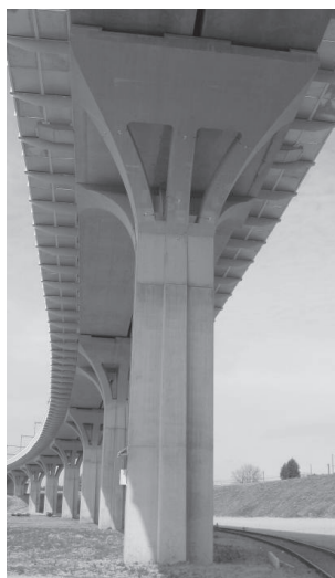
Fig. 1: Double track pier PA8 of the Iris railway viaduct
