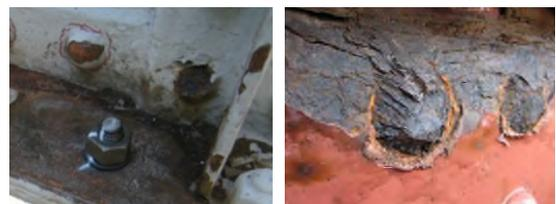
Figure 1. Rivet corrosion
