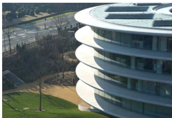
Figure 1. The building façade with the concrete sun-shading elements
