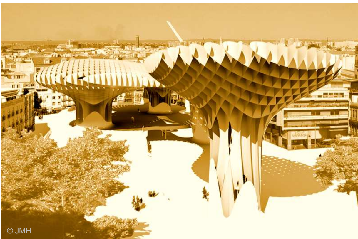
Fig. 1: LVL-Timber structure with 3 mm Polyurethane coating
