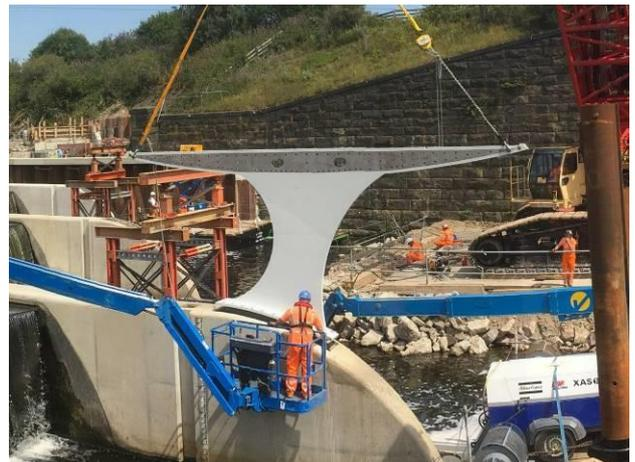
*Fig 3. Pier installation*
