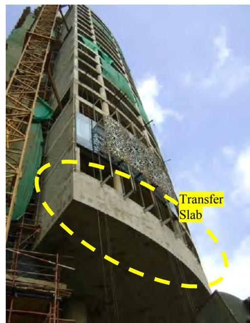
*Fig. 1: High-rise building with a transfer slab.*
