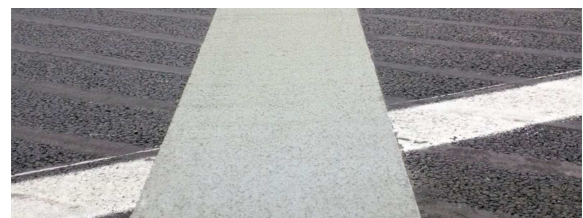
Figure 1. A Polyflex®Advanced expansion joint
