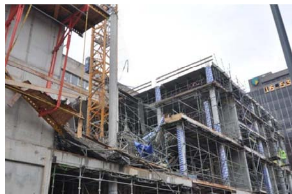
Figure 1: Collapse of temporary scaffold for construction of the floor of the B-tower
