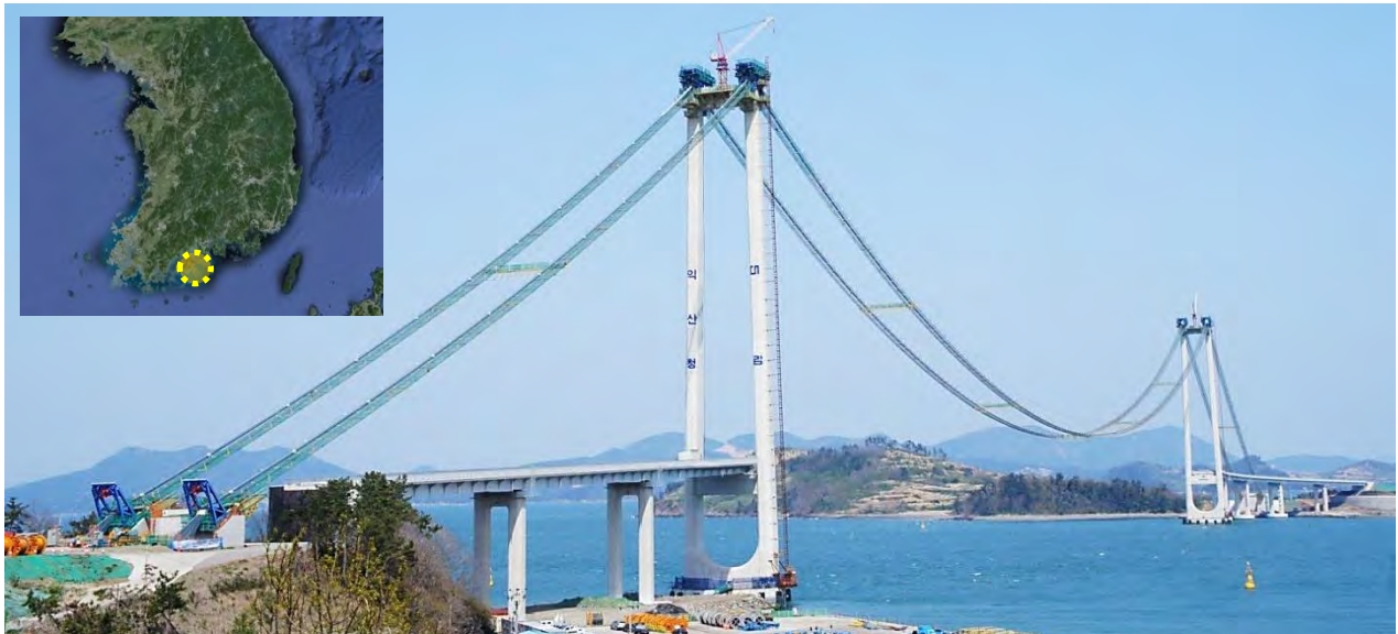
Fig. 1: The overall view of Jeokgeum Bridge after the completion of the cable erection
