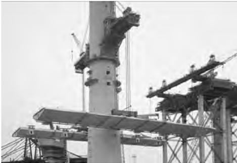
Fig. 2: Steel Deck Heavy Lift
