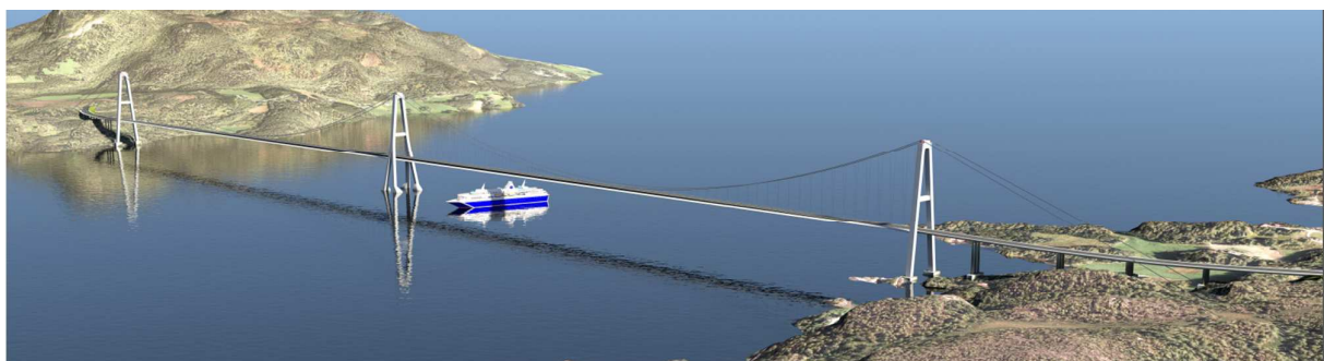
Figure 1. Overview of the bridge, shown with the 4-legged steel floater concept. Courtesy Arne Jørgen Myhre, Norwegian Public Road Administration.
