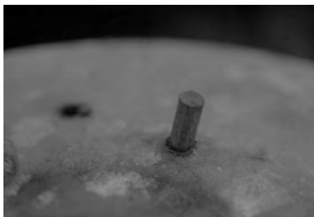
Fig. 2: Damaged anchorage protection cap
