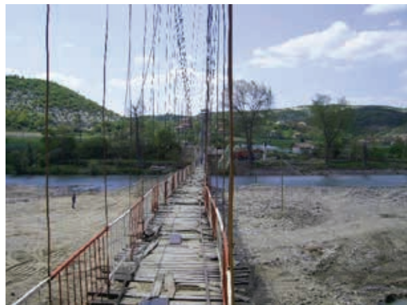
Figure 1: Bridge superstructure before the reconstruction
