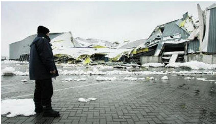
Fig. 1 *Industrial building collapsed due to snow load*
