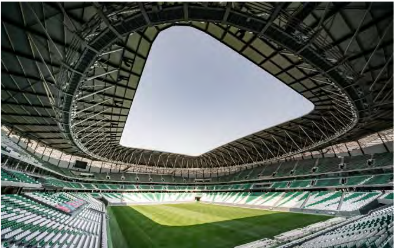
Figure 1. Internal photo of Education City Stadium showing the cable net roof
