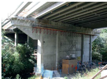
Fig. 2: Widened P3 cantilevers.
