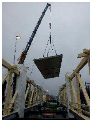
Fig. 2: Hoisting composite deck
