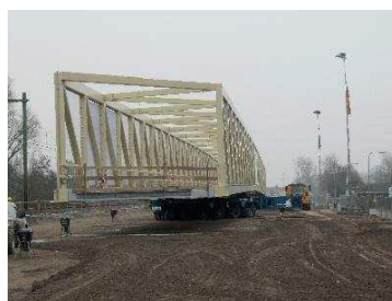
Fig. 1: Bridge on SPMT's
