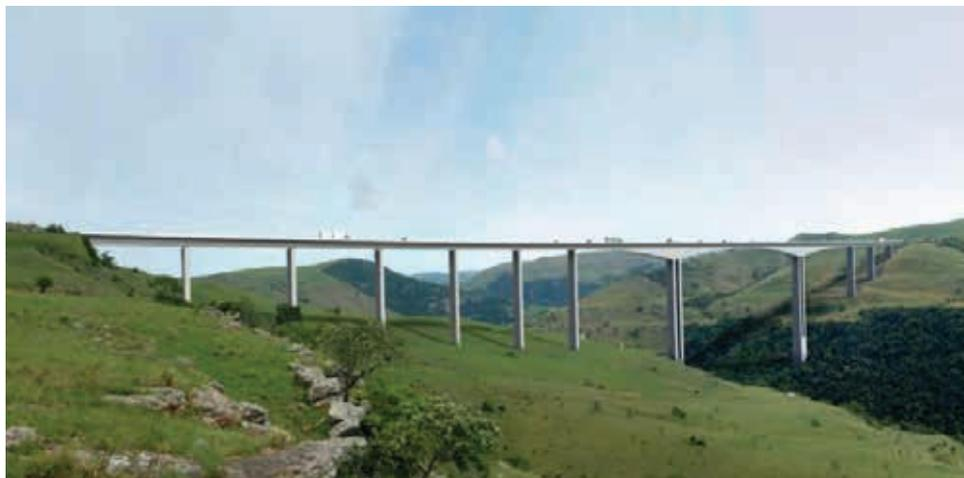
The main research topic: ILM applied on 66m span PC Beam without pile foundation
